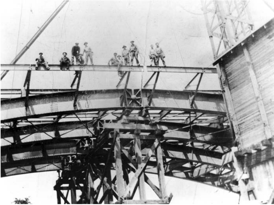
FIGURE 2. During the early decades of the twentieth century high-steel construction work became an increasingly important source of employment for men from Kahnawake. During the 1920s they were traveling to job sites throughout the Northeastern United States. Photo courtesy of the Kanien'kehá:ka Onkwawen:na Raotitiohkwa Cultural Center.
