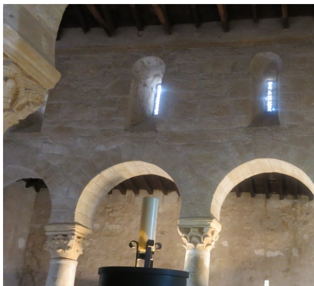
Fig. 22. Sprayed windows, San Juan de Banos, Spain
