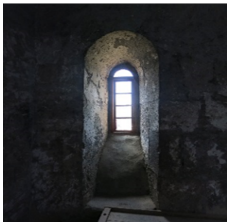
Fig. 21. Sprayed window, Mastara church, Armenia
