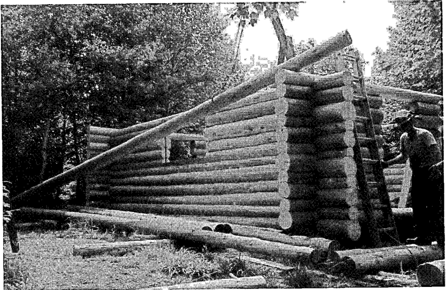
Fig. 10.3: Building "out of rounds" demands harmony between builder and nature.
