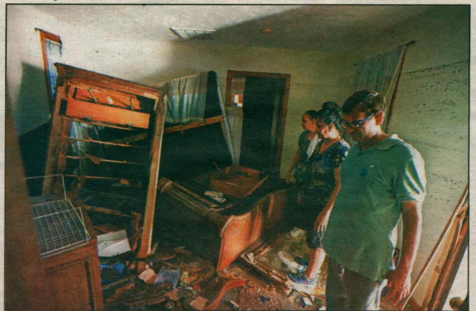
EXTENSIVE FLOODING ARE LEAVING THEIR MARK A WEEK AFTER HURRICANE FLORENCE HIT THE CAROLINAS. ASSOCIATED PRESS
