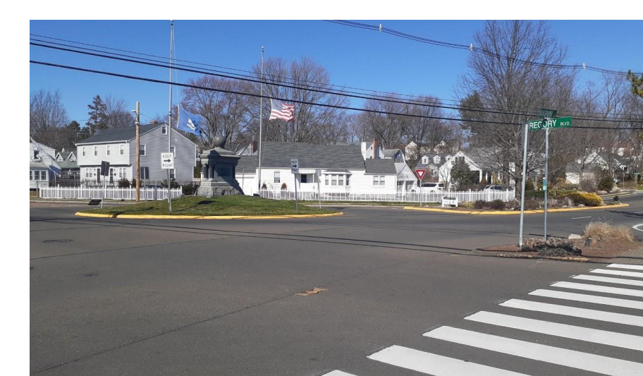
Fig. 5: Gregory Blvd Roundabout
